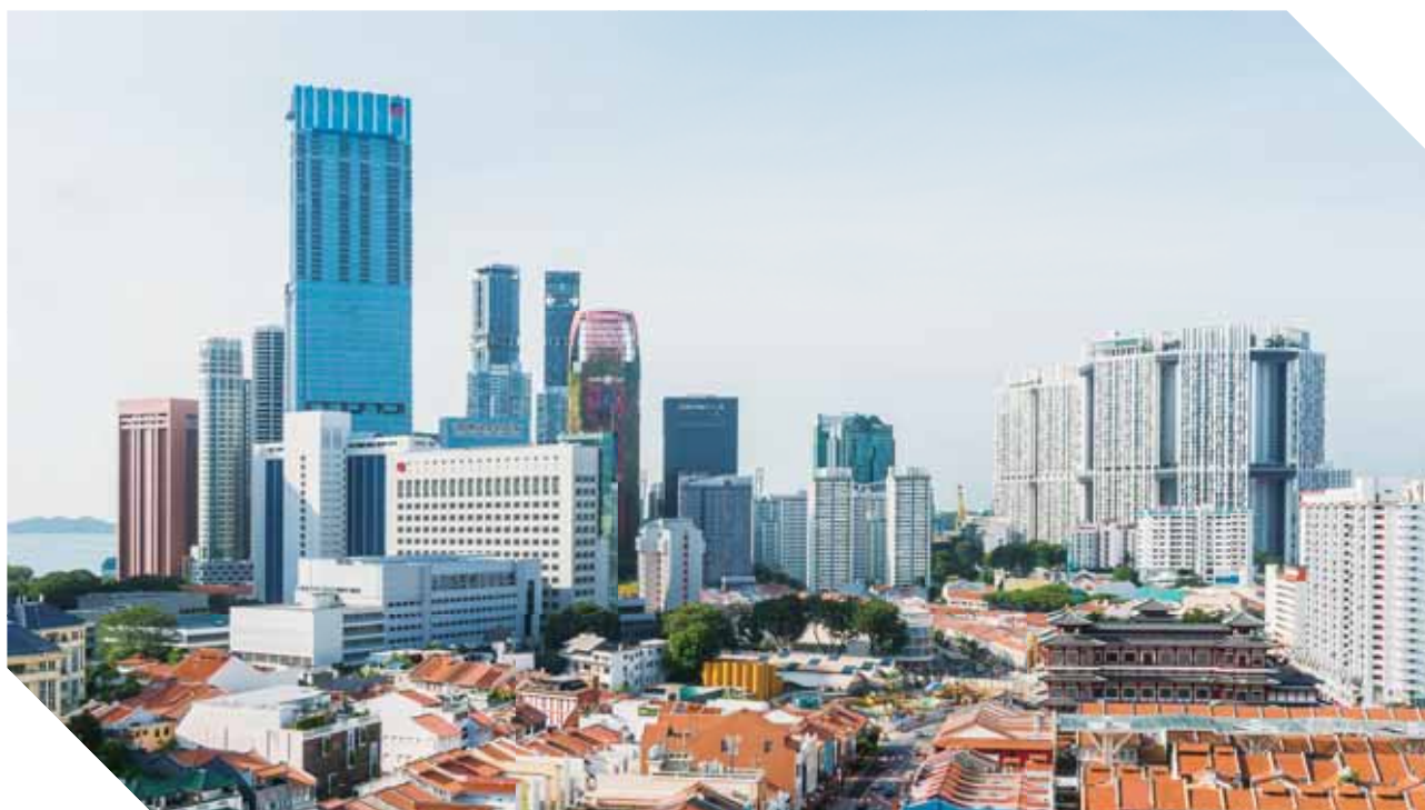
Tanjong Pagar Centre – currently the tallest building in Singapore
