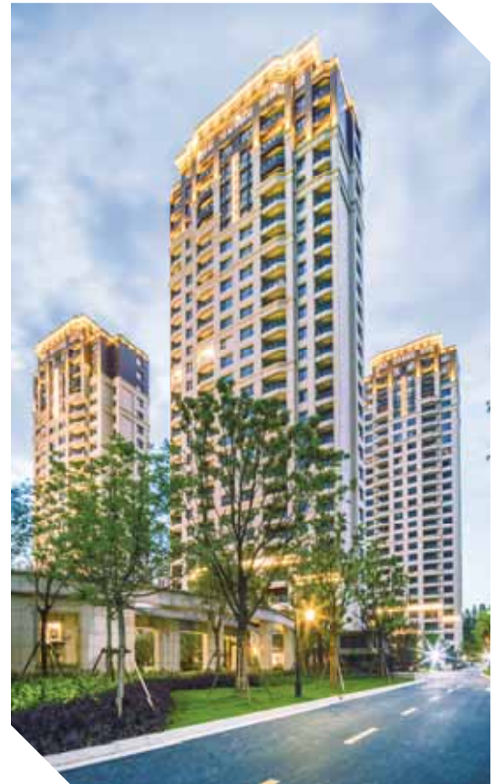
Exterior view of Changfeng Residence, Shanghai
